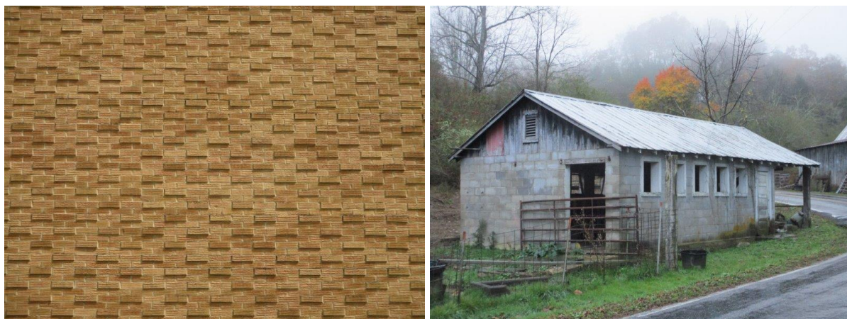
Silco Plant (detail) and the milking parlor at 124-143 Rocky Branch Road, Dillsboro vicinity.
