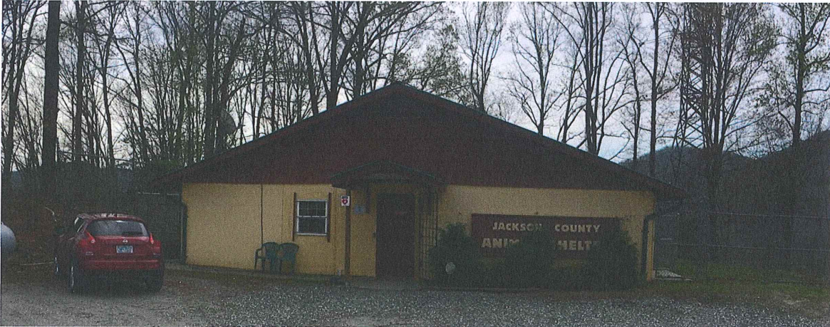
Photo above: Front elevation of the existing Jackson County Animal Shelter, Sylva, North Carolina
