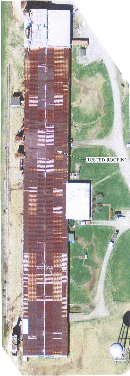
AERIAL VIEW OF ROOF 1" = 100'
