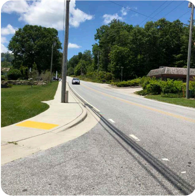
Image 19. This Cashiers Sidewalk has Been Designed Around Utility Poles to Maintain Sufficient Width for Wheelchair Users.
