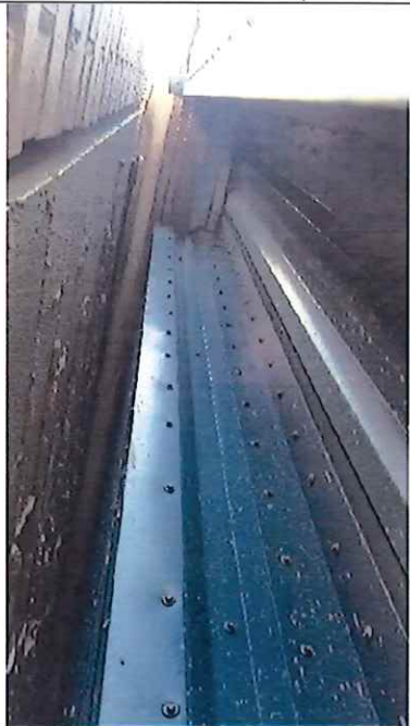
View into recess at existing building – insulation will be required under deck patch.
