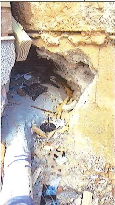
Roof leader tie-in at existing building – GC to patch corner of building.
