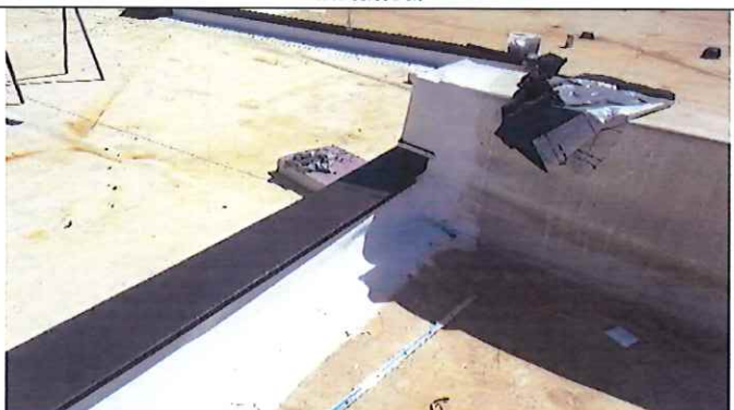
Roof expansion joint installed for majority of expansion joint.
