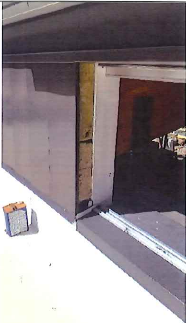
Kalwall - Sill flashing and bottom track installation – wrap sill flexible flashing up jamb of opening. Closure piece needed at jamb side – typical at locations with metal panel
