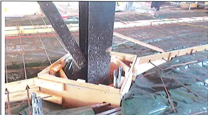
Columns at pool decks with concrete forms for column bases
