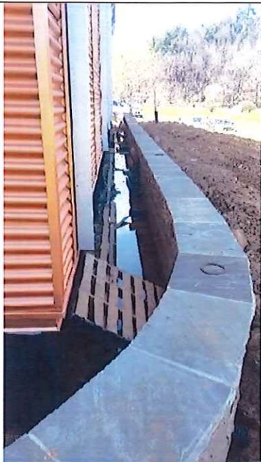
Planter area outside the leisure pool – storm drain tie-in in process. See previous field report notes about installation of insulation at foundation and tie-in of foundation drainage.
