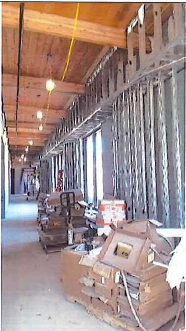
Dry corridor – curved wall framing and bench framing installed.
