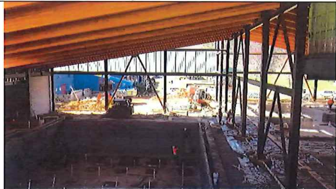
Competition pool – deck slab preparation in progress
