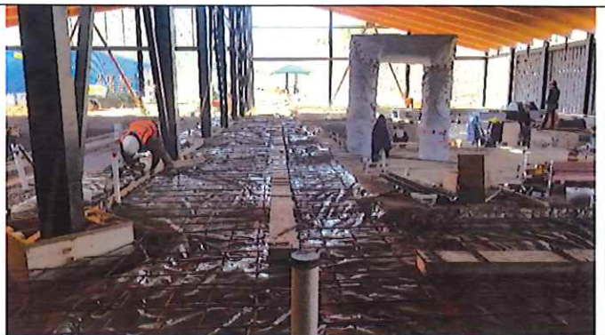
Leisure pool – deck slab preparations
