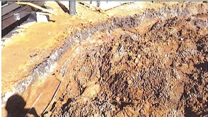
Grounding loop installation in trench
