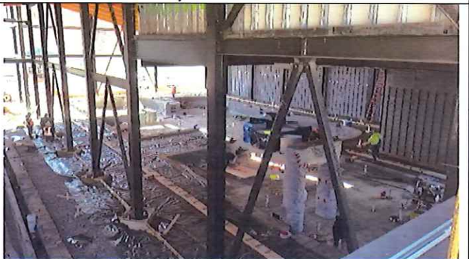
Leisure pool – deck slab preparation in progress
