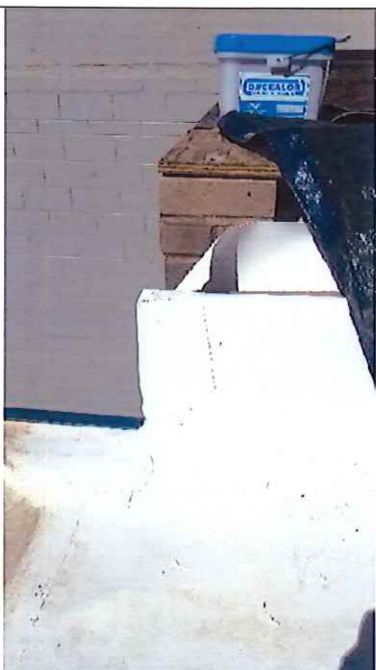
Roof expansion joint at recess area that required patch – see notes in field report
