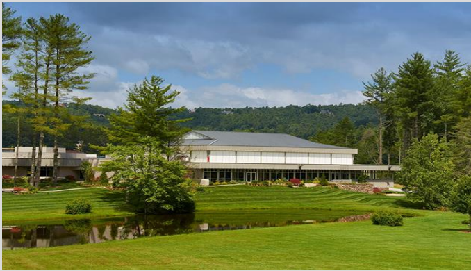
Pictured above is the Cashiers Recreation Center.
