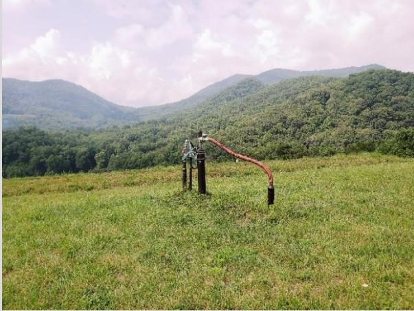
A Methane Gas Extraction Well Courtesy of the Green Energy Park
