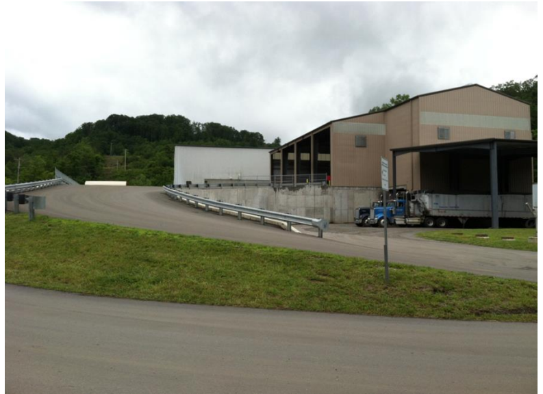
The Jackson County Transfer Station Courtesy of Public Works
