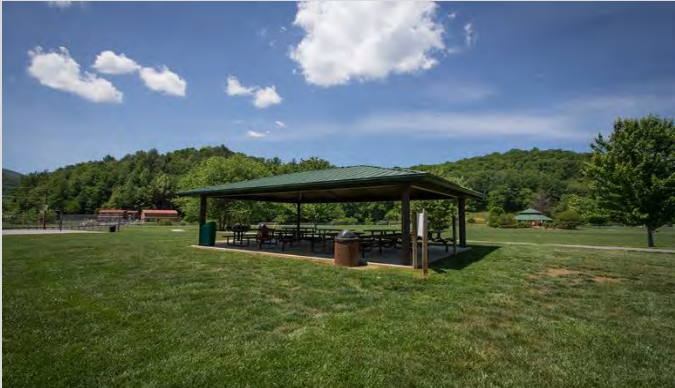
The Cullowhee Recreation Center Picnic Shelter.
