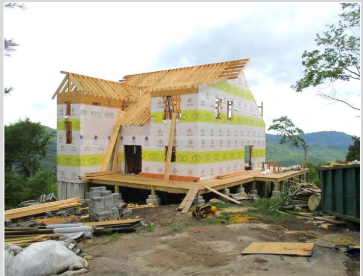
Residential Construction Site Courtesy of Permitting & Code Enforcement
